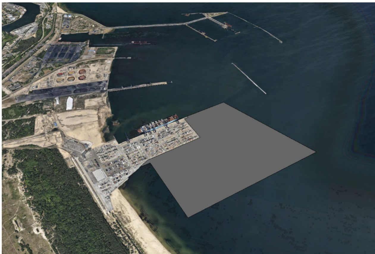
Figure 108 Visualization of the DCT berth transformation after the planned extension of the DCT3 terminal - bird's eye view from the east. Source: own compilation based on GoogleEarth
