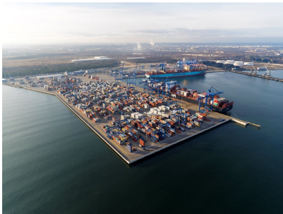
Figure 10: Water side view of the existing DCT terminal
