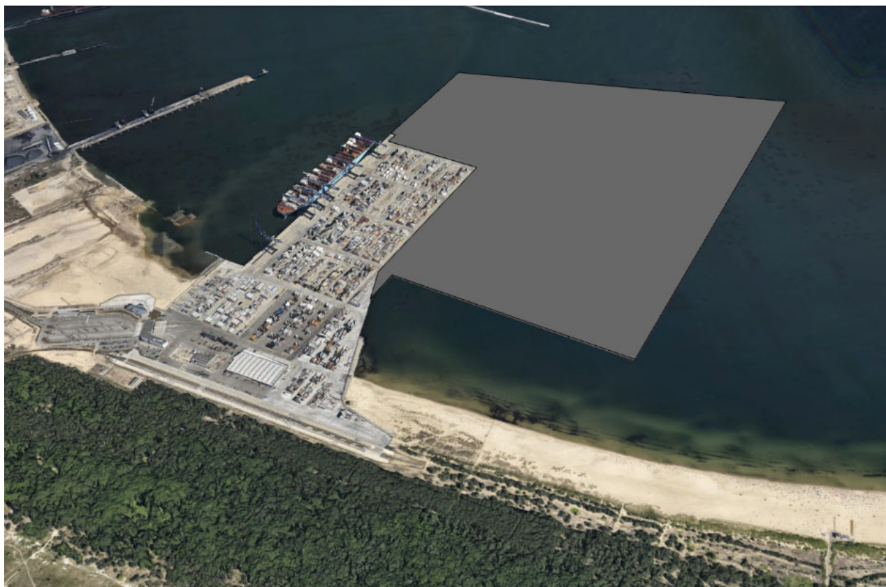
Figure 109 Visualization of the DCT berth transformation after the planned extension of the DCT3 terminal - bird's eye view from the southern side.
