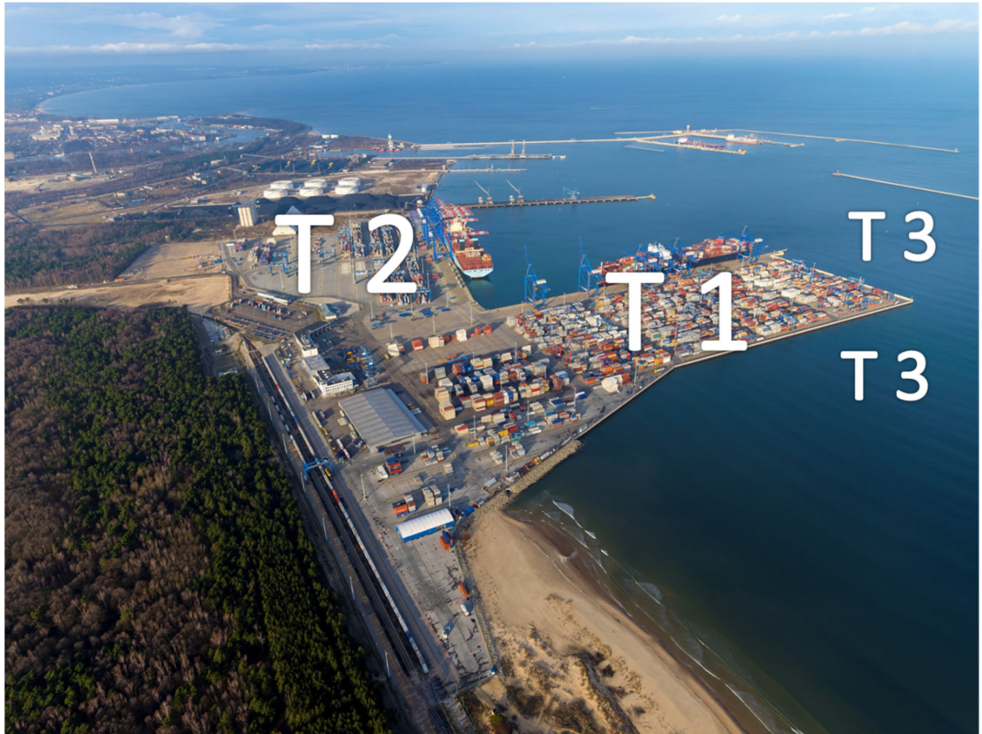
Figure 16: Location of T3 terminal in relation to existing terminals T1 and T2 - aerial photo Source: DCT/fot.aeromedia.pl
